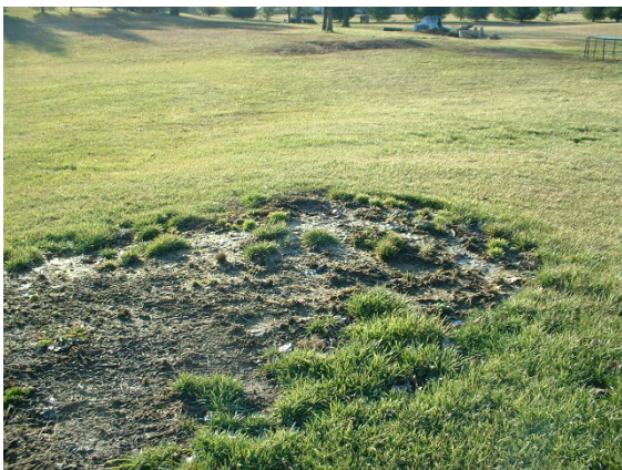
Failing drainfield. Photo by Todd Webb, REHS
